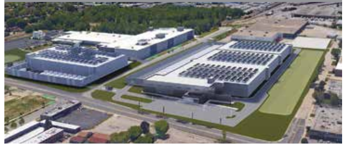
Below, a conceptual view of Digital Realty's planned expansion, which will increase the data firm's Franklin Park campus to 41 acres in area
