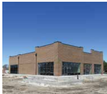
Construction on the Franklin Park Marketplace in 2017.
