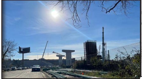
The Tollway began constructing the brand new I-490 Interchange.
