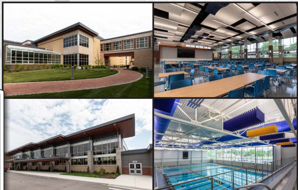
The expansion and renovations at East Leyden High School were completed. The combined renovation and addition projects cost approximately $90 million dollars. These projects are being funded without the need for a local property tax increase or a referendum.
