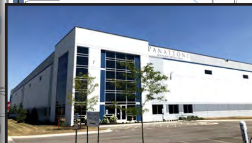
Pannatoni completes construction on a new 378,000 SF building at 11601 Copenhagen Ct.
