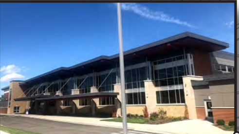
Construction continues on 122,00 SF expansion at East Leyden High School
