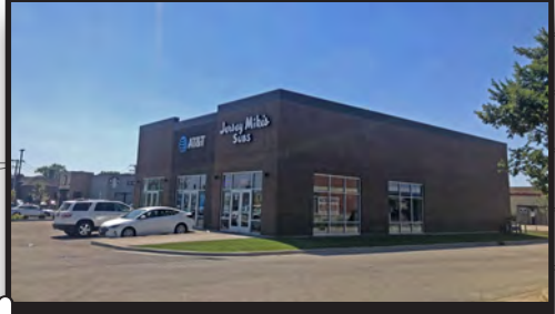
Glazier Development completes construction on a new retail building at 2830 Mannheim Rd.
