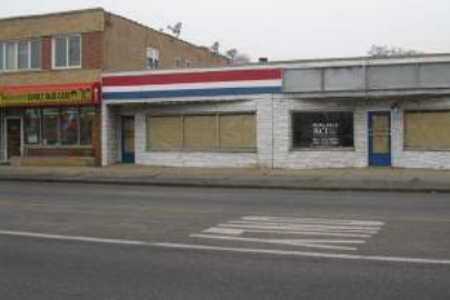
Commercial buildings along Grand Avenue
